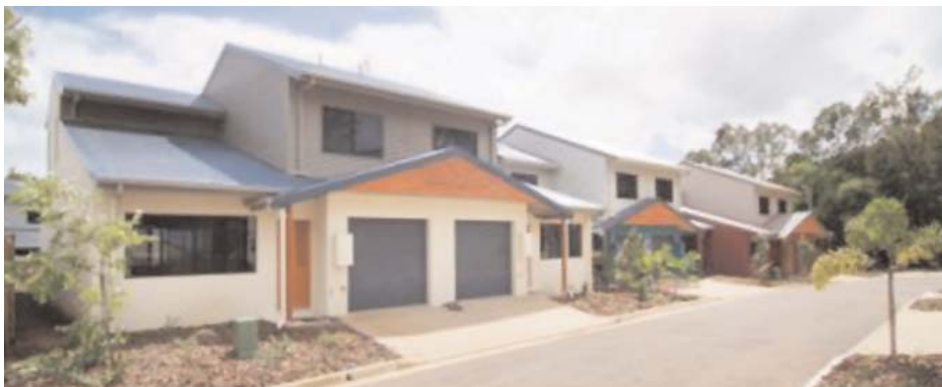
The Grove Development at Cannonvale
